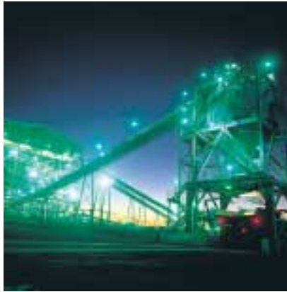
far left - Dragline operations at the Curragh mine, Qld
